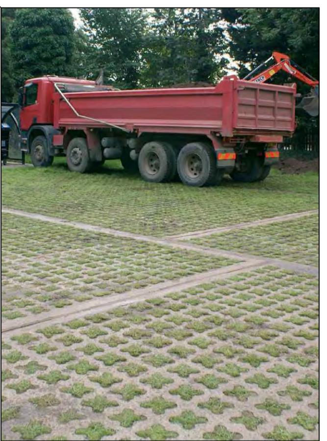
TYPICAL GRASSCRETE PAVING AFTER INSTALLATION
